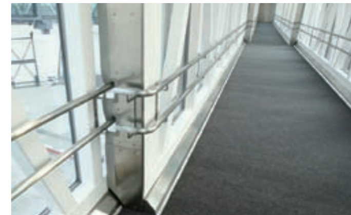
(Top) Floor gutters on both sides are hidden underneath the floor, making for a more spacious passageway. (Bottom) Universal design PBBs were the realization of a five-year dream for Mr. Saito.
