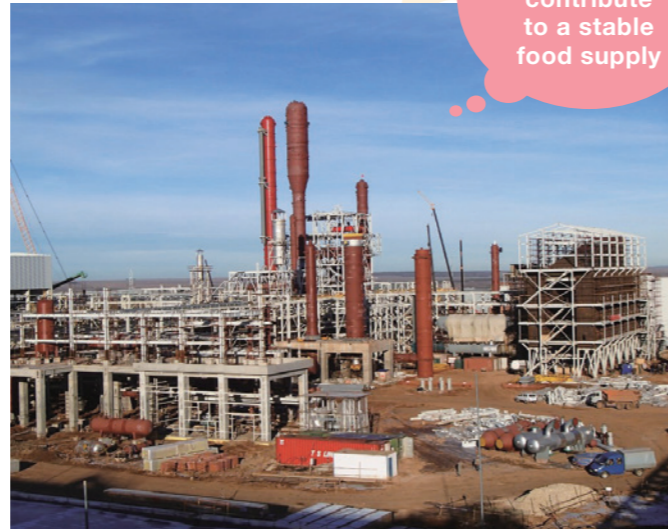
Fertilizer plant under construction in the Republic of Tatarstan (as of 2014)
