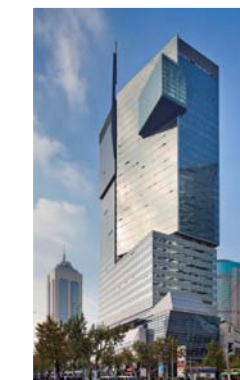
Gas Engine Distributed Power Generation Engineering Center (Shanghai, China)
