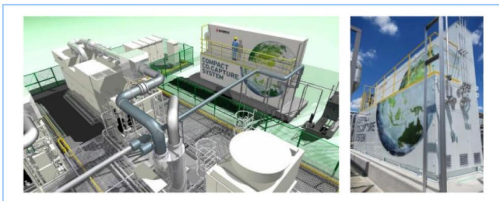
**Figure 8** 1,500kW power generation system using GS16R2 and compact CO<sub>2</sub> capture system
