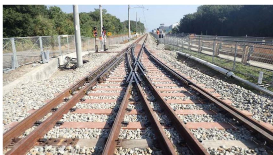
Figure 3 Dual gauge turnout
