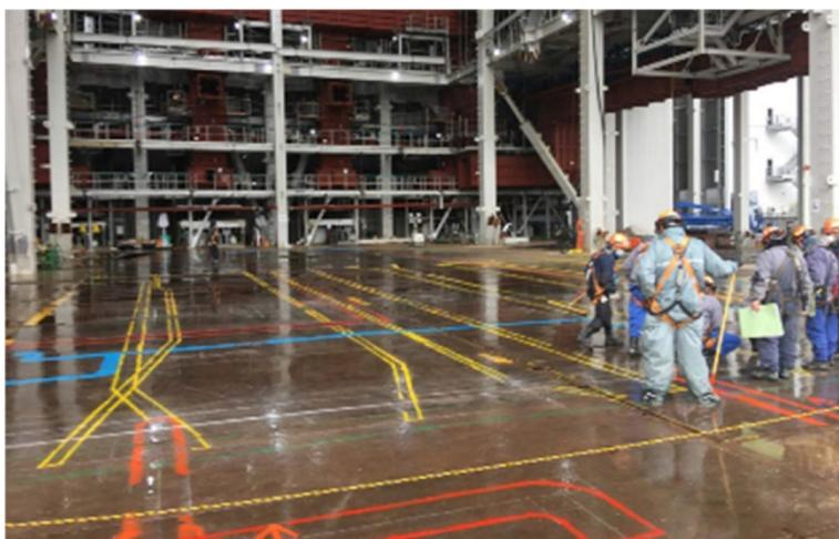
Figure 4 Markings for installation of equipment
