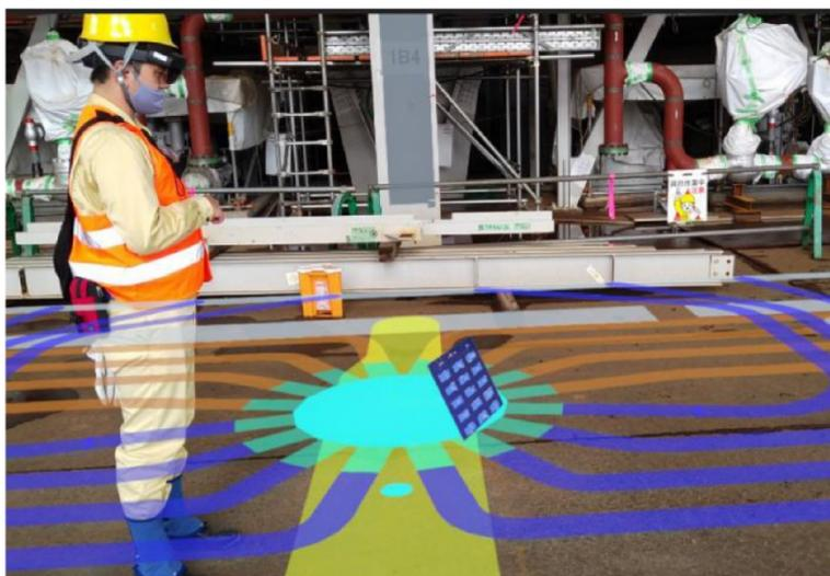
Figure 5 Superimposed display of marking positions
