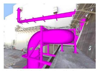
Figure 4 Graphic representation of 3D-CAD data superimposed on point cloud panoramic data
