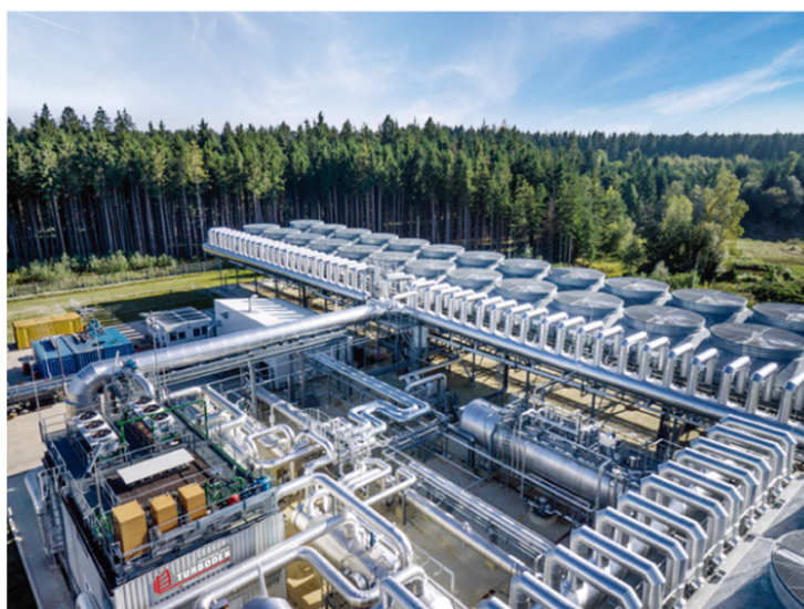
Figure 8 Existing binary plant in Germany
