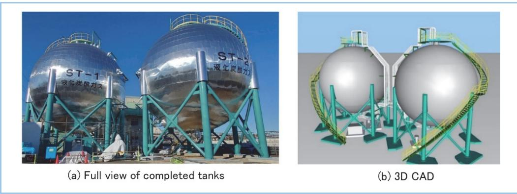
**Figure 2** Liquefied carbon dioxide tanks for Resonac Gas Products Corporation
