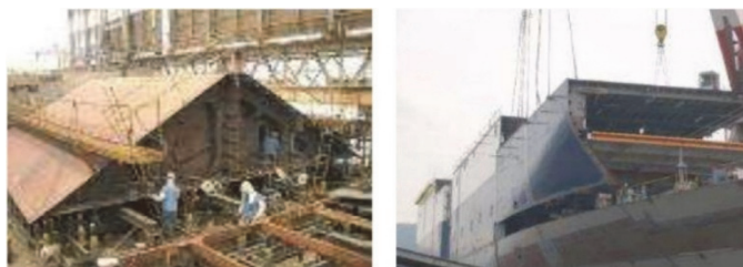
Figure 1 Blocks being assembled in shop (left) and being built in berth (right)
