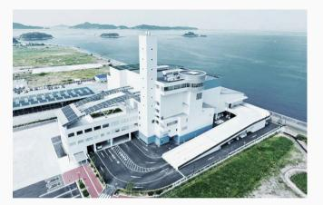
The Waste-to-Energy plants we developed safely incinerate and stabilize waste from general households and efectively utilize the extra heat from incineration for electric power.
