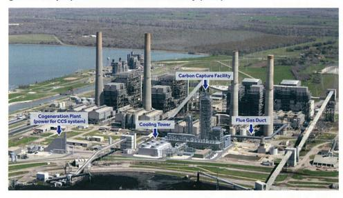
The capture system removes the carbon dioxide (CO<sub>2</sub>) from a slipstream of flue gas from an existing coal-fired power generation plant.
