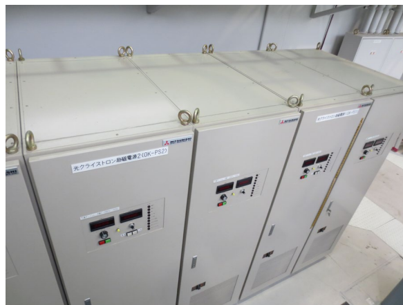
Excitation Power Source for Optical Klystron
