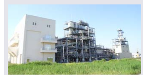
The largest plant in Japan: 200t/d
