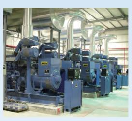
Whenever operating multiple generator sets in parallel, the prime mover and electrical systems should be protected to ensure stable load sharing characteristics, frequency stabilization, voltage stabilization and the synchronized closing of the circuit breaker.
