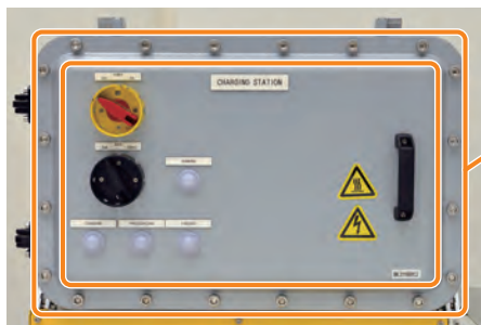
Joint surface between lid and enclosure
