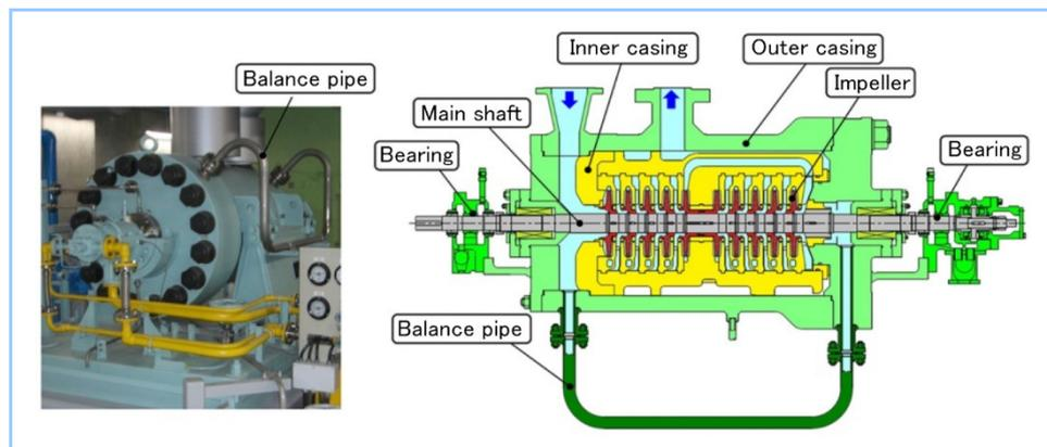
**Figure 7** High-pressure multi-stage pump for existing PWR plants
