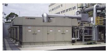
Fig. 4 The Advanced Miller GS16R-815kW hot water and steam recovery system in operation
