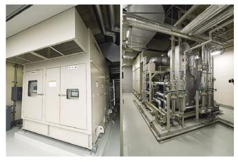
Fig. 6 The Advanced Miller GS6R-305kW hot water recovery system in operation
