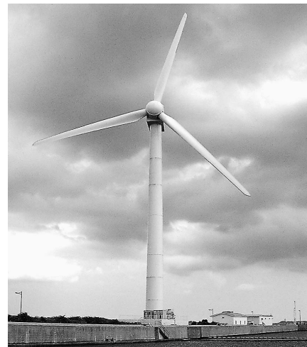
Fig. 11 Japan's first 2 000 kW wind turbine (MWT-S2000 at Gushikawa Power Station, Okinawa New Energy Development Co.)
