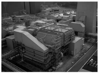
**Fig. 1 Flue gas treatment facility** Flue gas treatment facility at Unit 1 of the Tachibana Wan Power Station of the Electric Power Development Co., Ltd.; 1 050 MW, the largest capacity coal fired power generation plant in Japan; A single tower type absorber (double-contact flow scrubber); Desulfurization efficiency 95%
