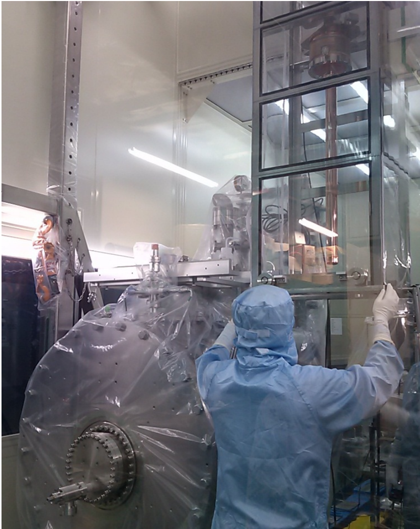
Installation of Power Coupler at NSRRC
