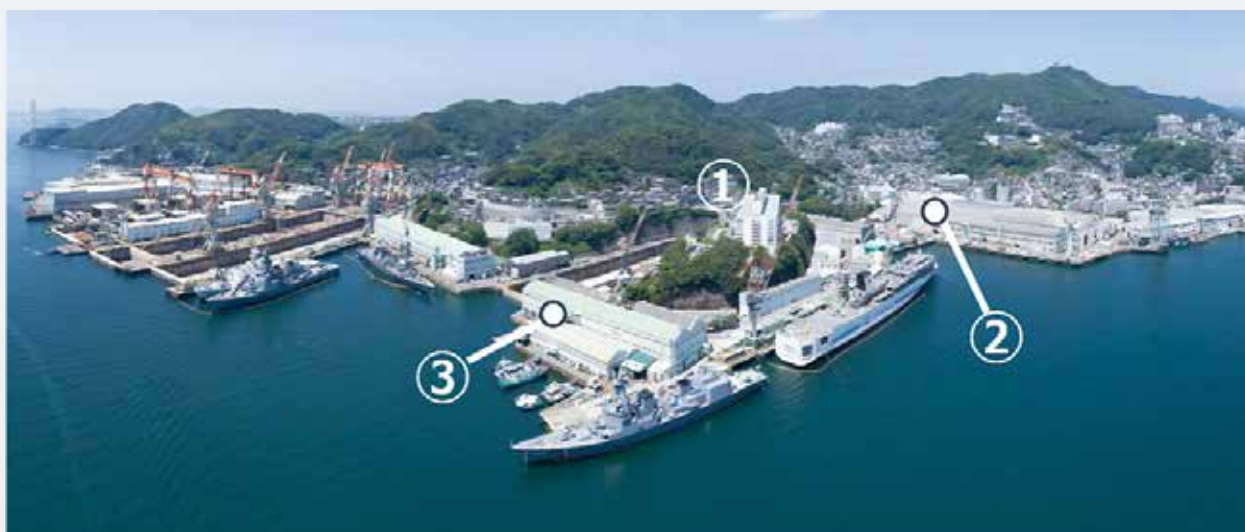
①Office ②Parts Center ③Turbocharger Shop
