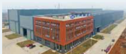
Panoramic view of new factory
