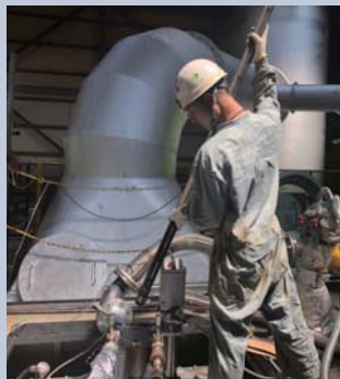
Installing a combustion equipment sprayer
