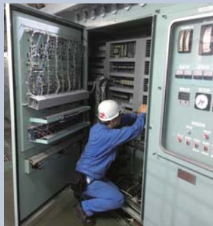
Modifying a control system panel
