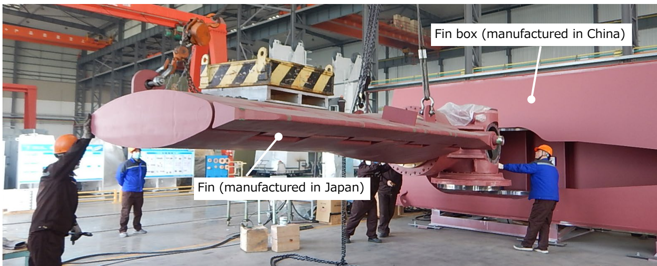
Fin stabilizer assembly operation scene
