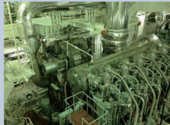
As installed on the bulk carrier
