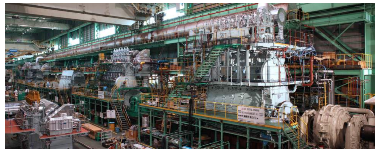
Inside the Plant
