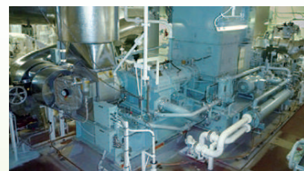
MERS power generator installed on the ore carrier
