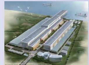
QMD Plant (Qingdao, Shandong Province)
