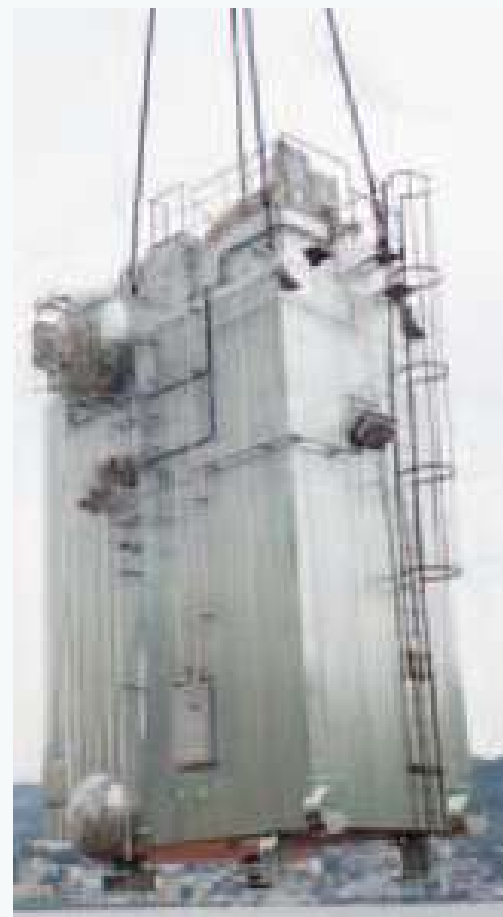
A regas boiler being loaded onto a ship
