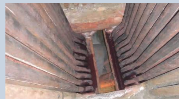
Superheater tube replacement work
