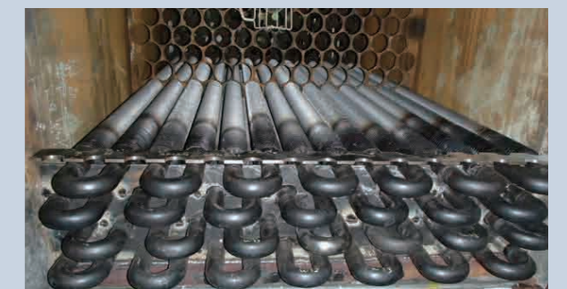
Economizer tube replacement work
