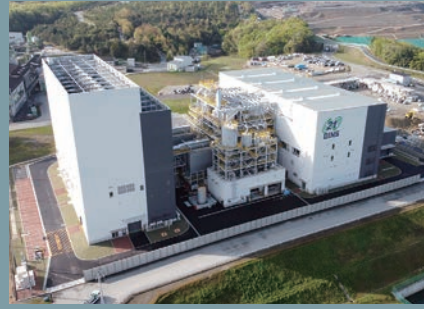
Industrial Waste-to-Energy Plant
