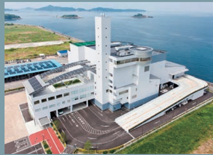
Municipal Solid Waste-to-Energy Plant
