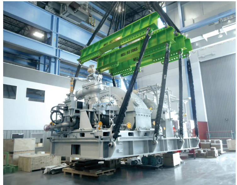
Complete packaging of two steam turbines and one compressor package for a critical footprint replacement project lifted on our 300-ton capacity bridge crane.
