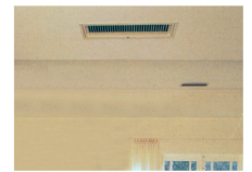
FDUM Duct Connected type
