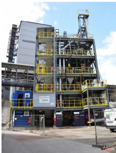
Photo of the HYFOR direct reduction pilot plant for iron ore fines developed by Primetals Technologies and located at the voestalpine site in Donawitz, Austria. The DR process is CO 2 -free and H 2 -based
