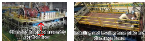
Photos of Changeover Process
