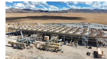
Geothermal power plant site in U.S.
