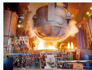
Large electric arc furnace (EAF Ultimate)
