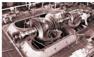
Mitsubishi Westinghouse turbine
