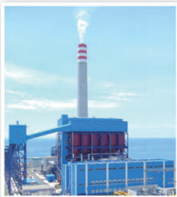
▲ Paiton III Thermal Power Plant
