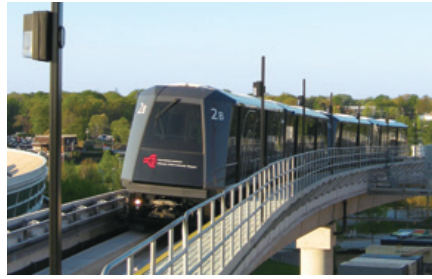
Automated People Mover (Crystal Mover) for Hartsfield-Jackson Atlanta International Airport
