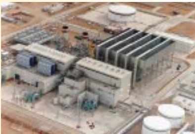
Chihuahua Combined Cycle Power Plant (Mexico)
