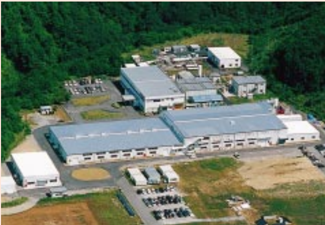
Solar Cell Production Plant
