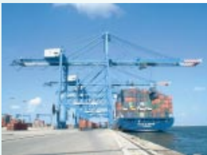
Container Handling Quayside Crane
