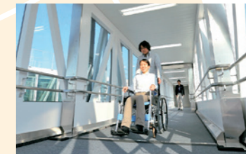
No more ups and downs; wheelchairs and strollers roll smoothly along the corridor.
