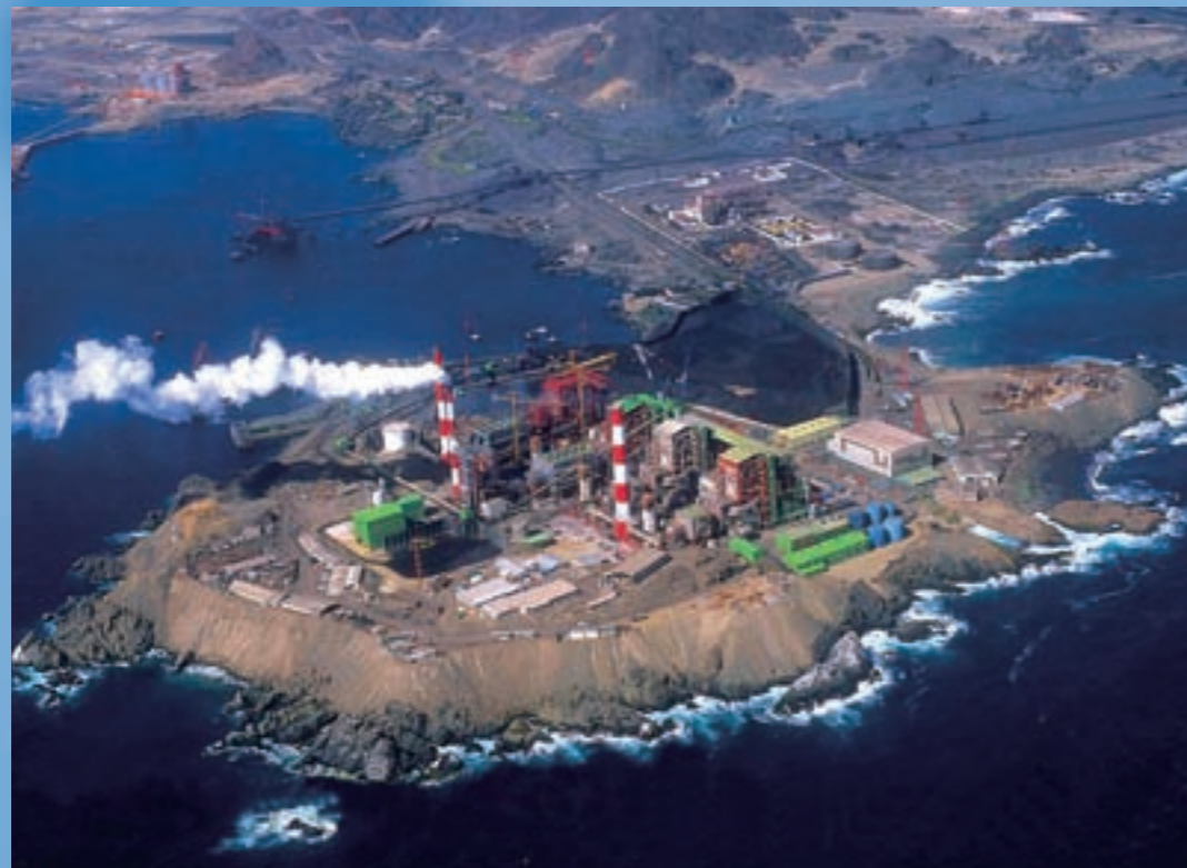
Construction work underway on the No. 4 unit. The construction site was on an extremely hard bed of rock – a hurdle for the foundation work that had to be overcome by means of construction blasting.
