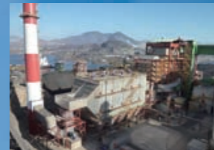
The No. 4 unit is equipped with SCR system that meets Chile's environmental regulations. It is the first coal-fired power plant with this in the country.
