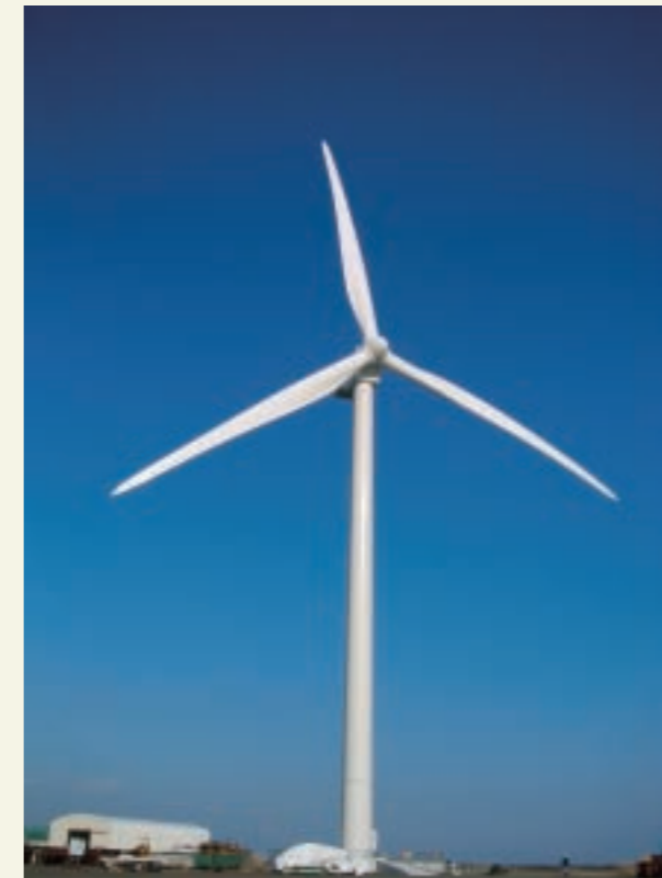
Wind Turbine (image)
