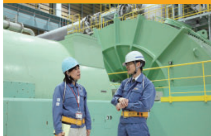
(Top) Mr. Akiyama explained how "water is changed into steam by heat from the nuclear reactor, and that steam rotates the turbine to generate electricity." (Bottom) In front of a steam turbine with 54-inch blades, among the largest class blades in Japan.
