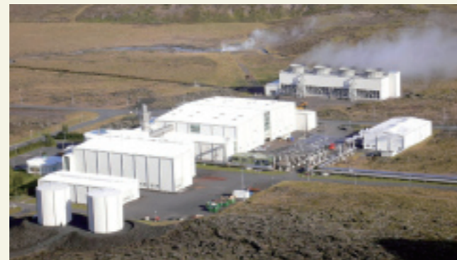
Geothermal power plant
