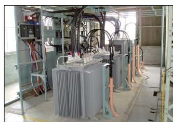
Energy-saving distribution transmitters
