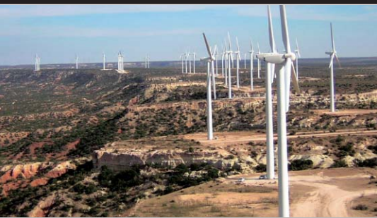
Wind farm (Texas, USA)
