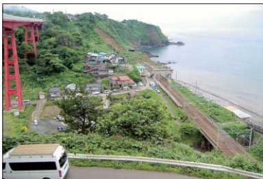
Investigation with priority given to bridges that were heavily damaged
