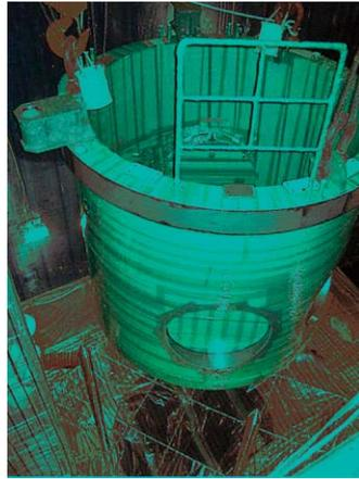
Fig. 8 Installation shielded platform in R/V
