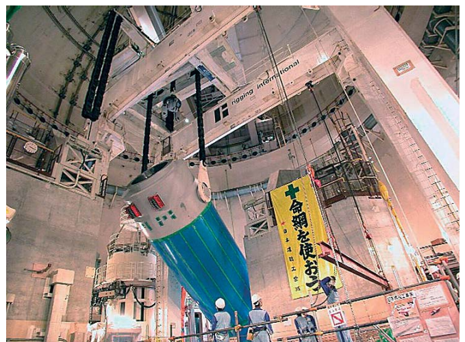
Fig. 2 The special crane and the storage cask in the reactor containment vessel
