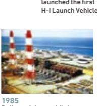
1985 Delivered the world's largest combined cycle power plant, Tohoku Electric Power Higashi Niigata Plant Unit 3, No. 2 Series (545 MW)
