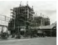
1968 Completed the first domestically produced 500 MW supercritical pressure boiler, Chubu Electric Power Chita Thermal Power Station Unit 3 (1,700 t/h)
