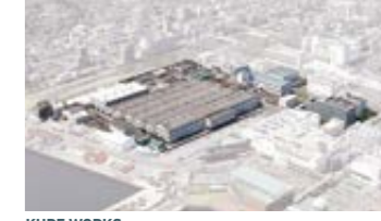
KURE WORKS ■ Energy Systems
